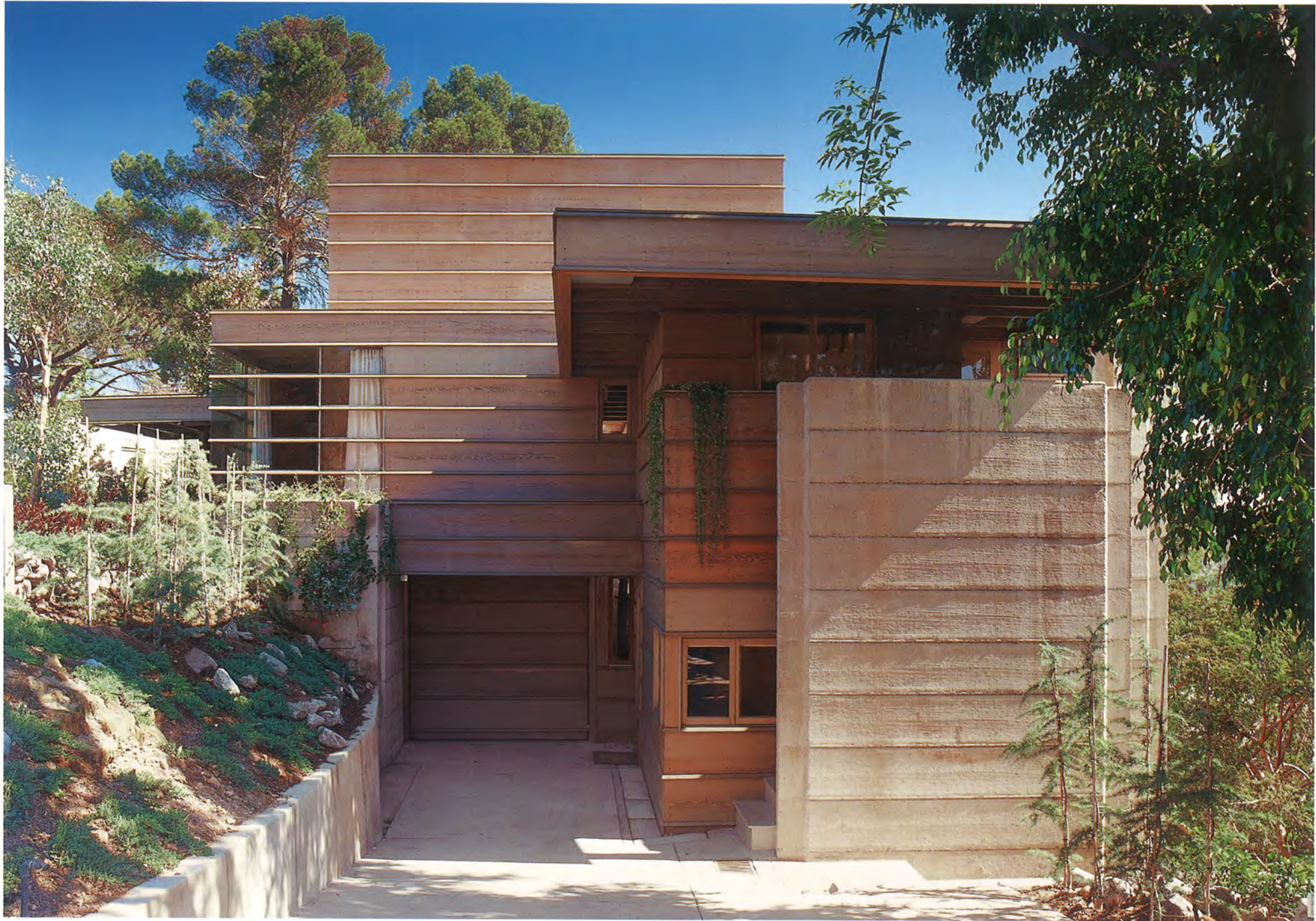
ABOVE: Front elevation with garage; the kitchen wing is to the right. The 16-inch horizontal module expressed in the shuttering concrete substructure is echoed in the wood banding above. OPPOSITE: The dining room with reproduction Rudolph Schindler furniture.
